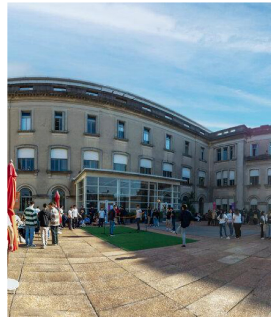
Figure 1. The CORE Center facilities at the Universidad Católica de Uruguay.
